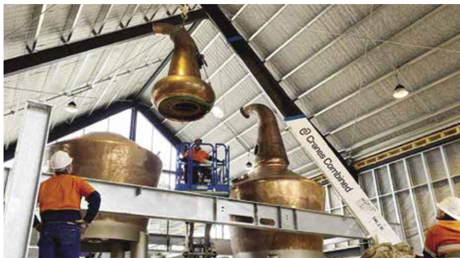
In recent weeks the distillery took delivery of two custom made copper pot stills, fabricated by Stillsmiths Tasmania in Westbury.
